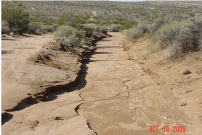
Figure 4. New downcutting on OHV trail after rains.
