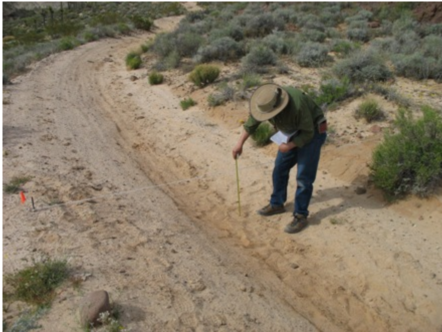
Figure 3. A long tape measure was extended between the two spikes and depth measures were taken at one-foot intervals within the roadway. A profile of the road surface is thus produced, and measurements of soil loss can be calculated using the recorded figures.
